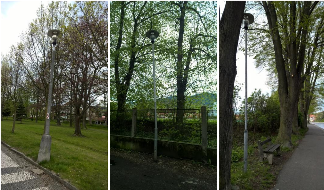
Fig. 30. Town of Sušice, The example of obsolete pole, all installed lamps have no arm and are mostly shaded by trees
