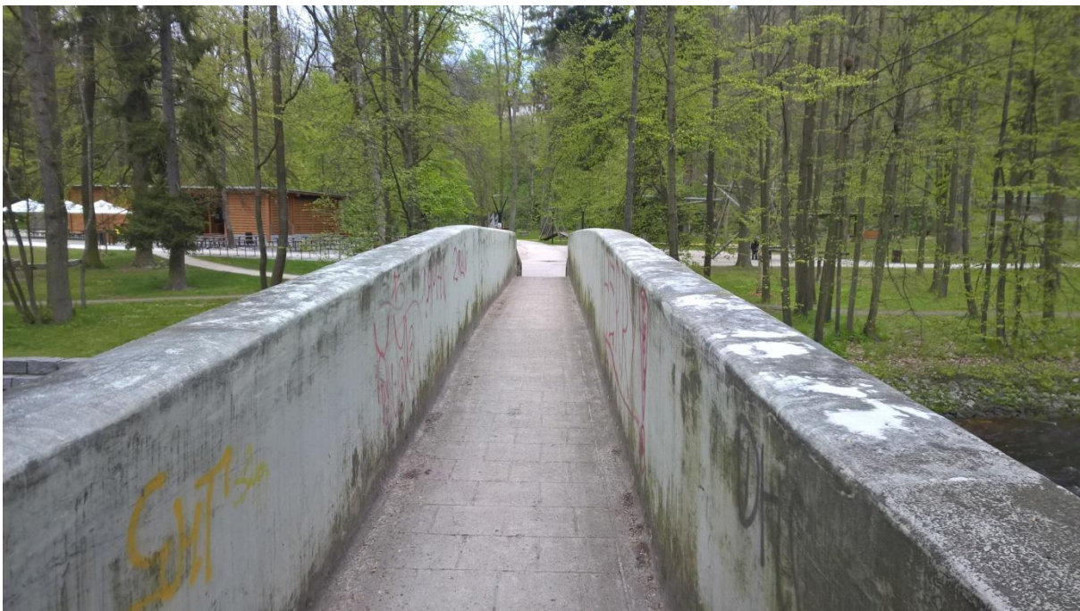
Fig. 20, Town of Sušice, Bridge connecting Santos with island
