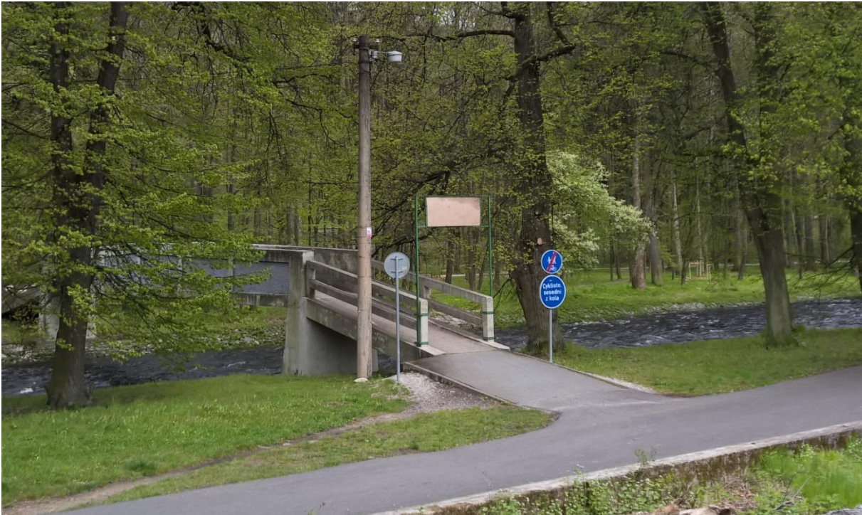
Fig. 20, Town of Sušice, The detail of aged luminaire which provides the illumination of the bridge
