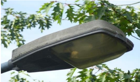
Typical technical luminaire with 50 W HPS lamps
